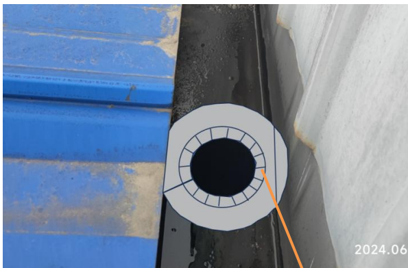
Treatment around rainwater bucket
