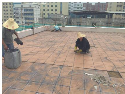
Repairing roof tiles
