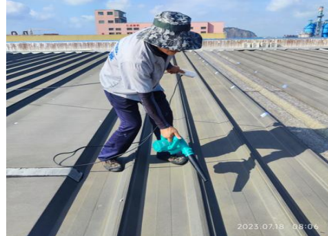
Blower to remove the dust
