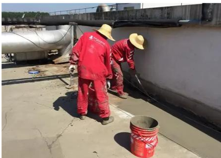
Filling with cement mortar
