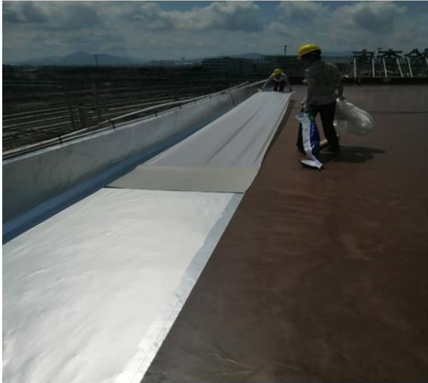
Lay the first piece from the bottom
