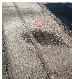
Remove loose shale gravel
