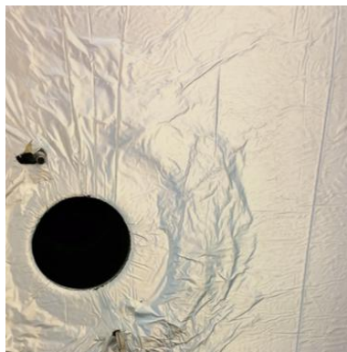
Cut off the membrane around the drain outlet
