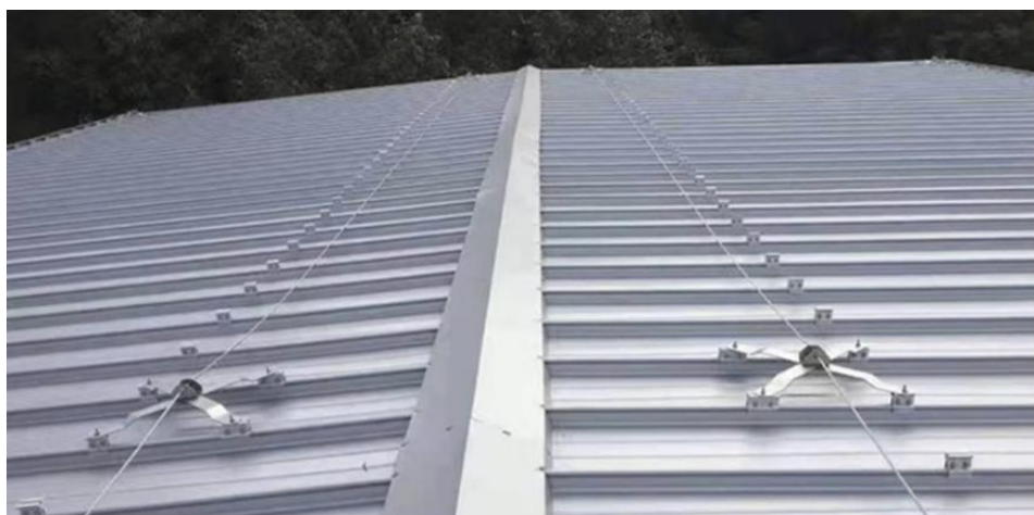
Anchor bolts and safety cables
