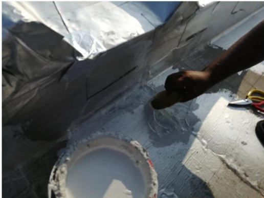
Treatment of joints in the gutter
