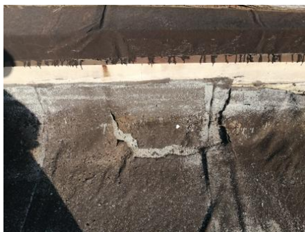
Shoveling away aged SBS membrane
