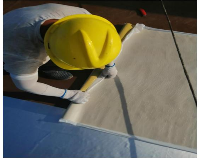
The upper roll covers the lower one
