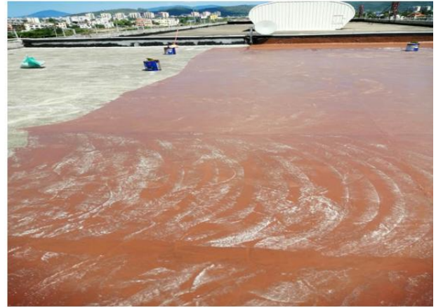
Apply polyurethane paint
