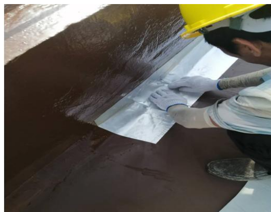
Additional layer to inner corners
