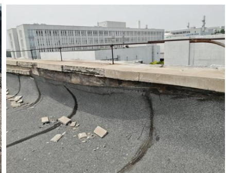
Peel off aged parapet veneer
