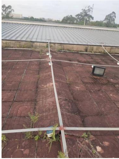
Clean up weeds and loose bricks from the
